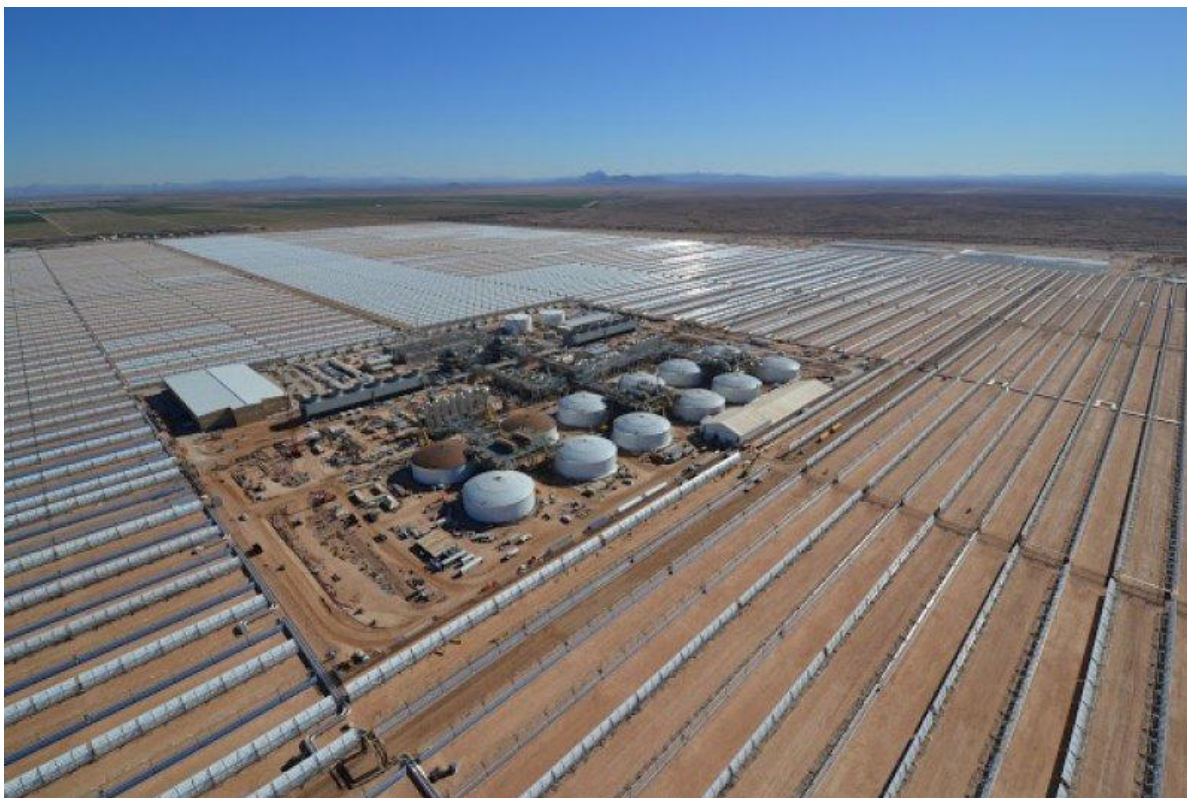
Figura 24 – Usina termosolar Solana (280 MW) com 6 pares de tanques de armazenamento. (Fonte: http://www.csp-world.com/news/20131004/001211/arizona-utility-highlights-benefits-csp-plants-energy-storage )
